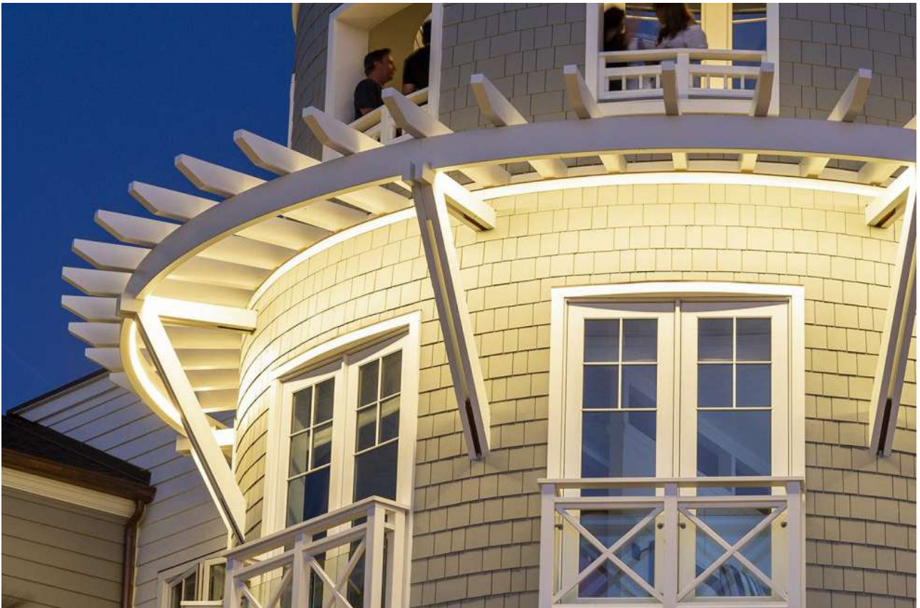
Lido House Hotel – Newport Beach, CA. - Lighting Design First Circle Design Architectural Design: WATG Photos: ©SAC Design
