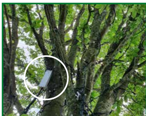
Placing the driver in the crown of the tree is the safest solution (e.g. in public areas)
