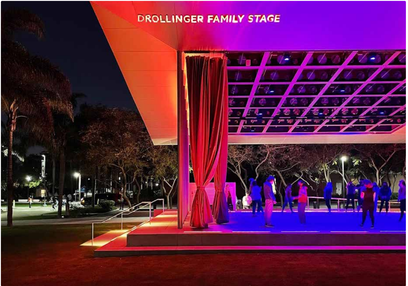
Colour mixing of RGBW fixtures is managed by DMX RDM drivers.
