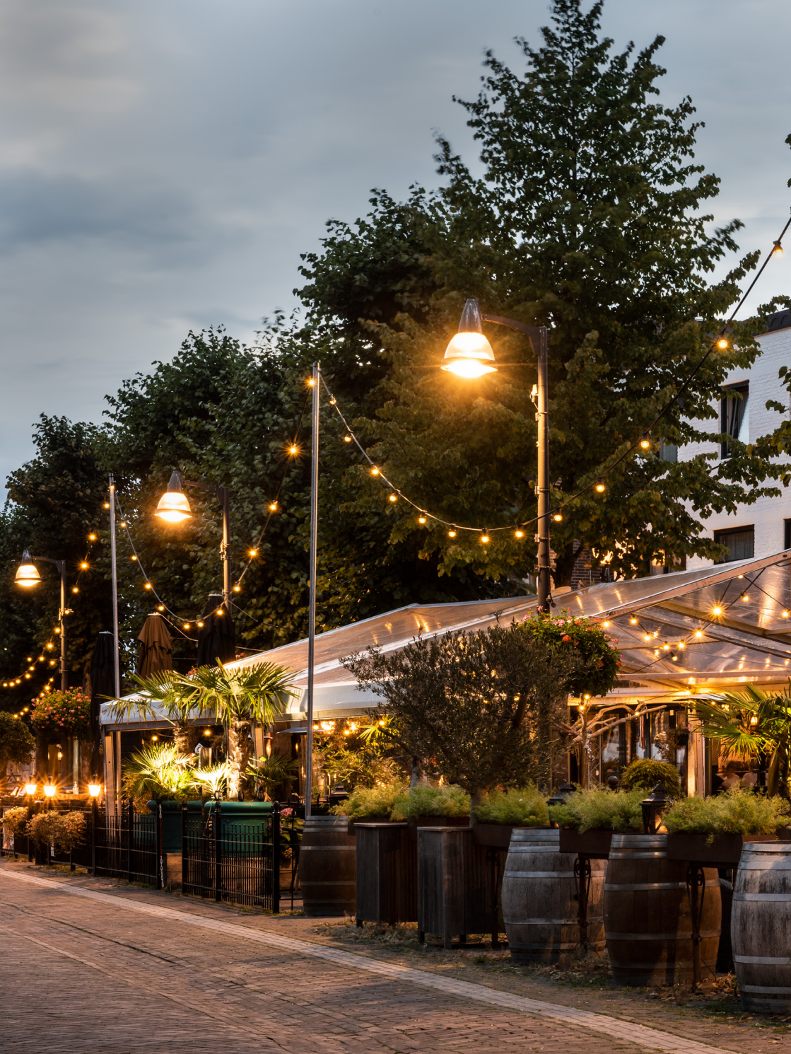
Festoon Cable Light at atmospheric street 'de Preek' - Uden, the Netherlands
