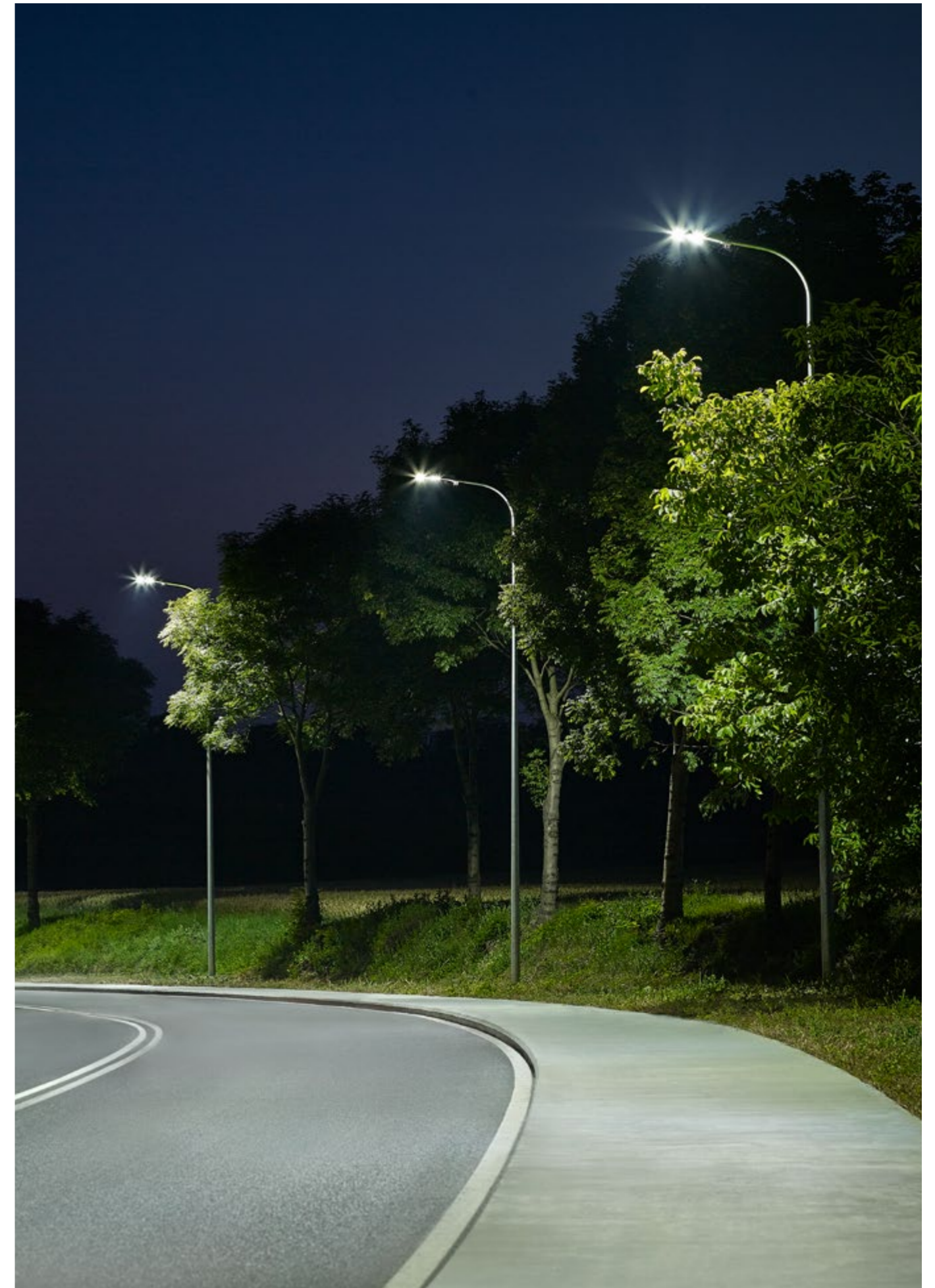
Application of Corona Street LED Evo 2 in Środa Wielkopolska.
